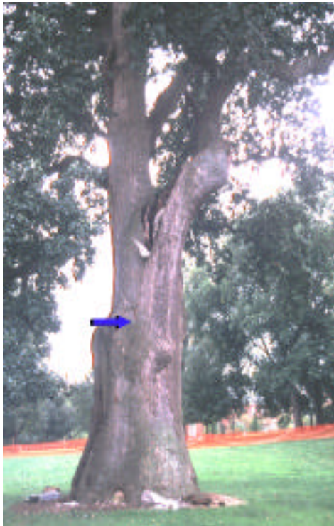
Figure 3 View from the north, showing location of the bottom of the crack (blue arrow).
